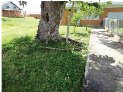
(Left Photo) Remove tree and surface roots and reconstruct concrete walkway.
