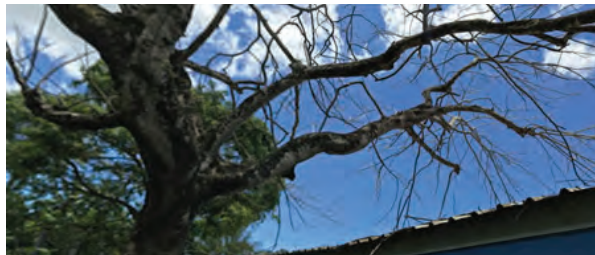
Figure 27: Example of a large dead tree with branches overhanging a classroom building.
