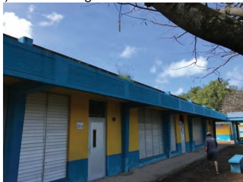
Remove debris and vegetation growing within the rain gutters and flush out downspouts to drain. Repair or replace sections of rain gutters as necessary.
