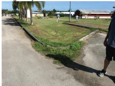
(Left Photo) Rake and remove grass clippings after cutting to prevent clogging of swales and drain inlets.
