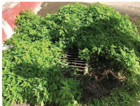
Remove overgrown grass / weeds covering major drain inlets and remove dirt and debris inside the drain inlets and flush drain lines.
