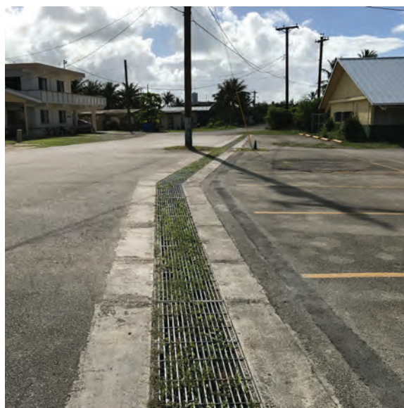
Figure 2: Trench Drain
