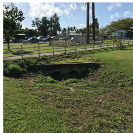
Figure 5: Drain Pipe Headwall
