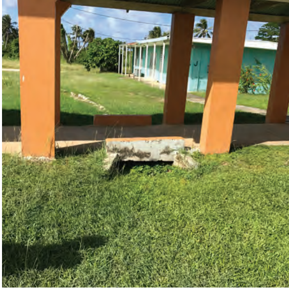
Figure 6: Sidewalk Culvert
